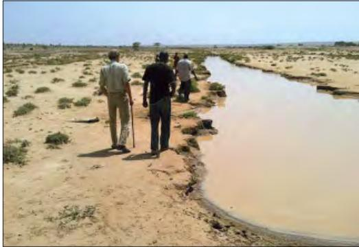
Fig. 14. Kenya: retaining water in dry areas by making contour trenches (Photo: Naga Foundation).
